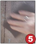
Sand or rub of all excess media, MUST be painted with topcoat, we suggest Latex based, high endurance, high traffic paint coatings
