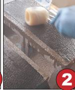
Roll HM180C3P topcoat providing ample coating and make sure is wet
